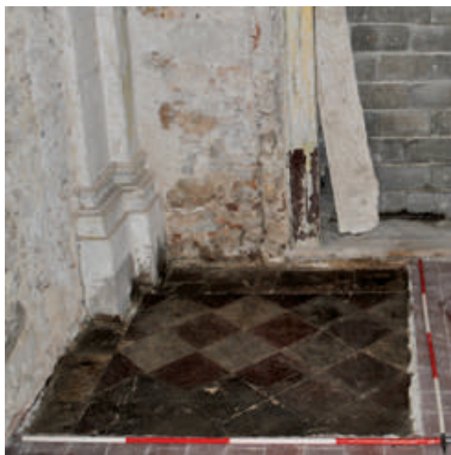
6. Barokno popločenje u sjevernom kutu crkve sv. Nikole / The Baroque period paving in the north corner of the St Nicholas church (foto: Š. Vrkić)
